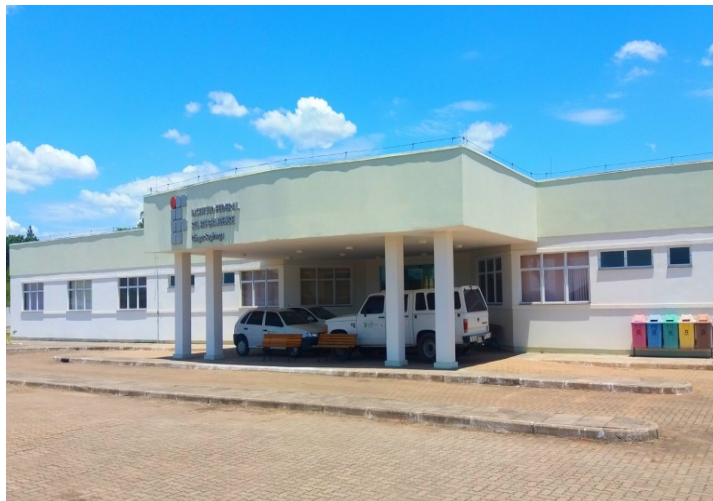
Figura 3 – Bloco multifuncional do IFSul, campus Sapiranga
